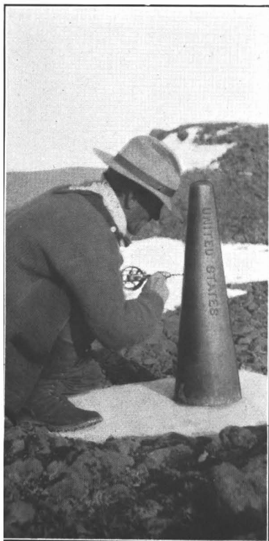
Type of small monument, and method of numbering. See page 192.
