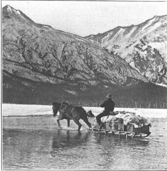
Crossing the Chitina River. This sled is placed on another temporary sled to keep the load above water.
