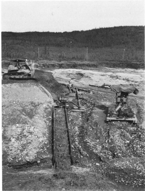
FIGURE 12 Bulldozer sluing operation on Dominion Creek.
