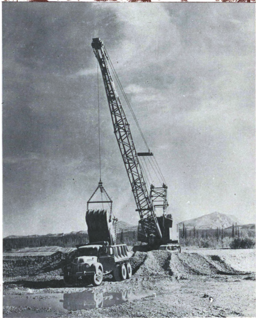
Gravel for the pipe-line road being loaded into truck by drag-line.
