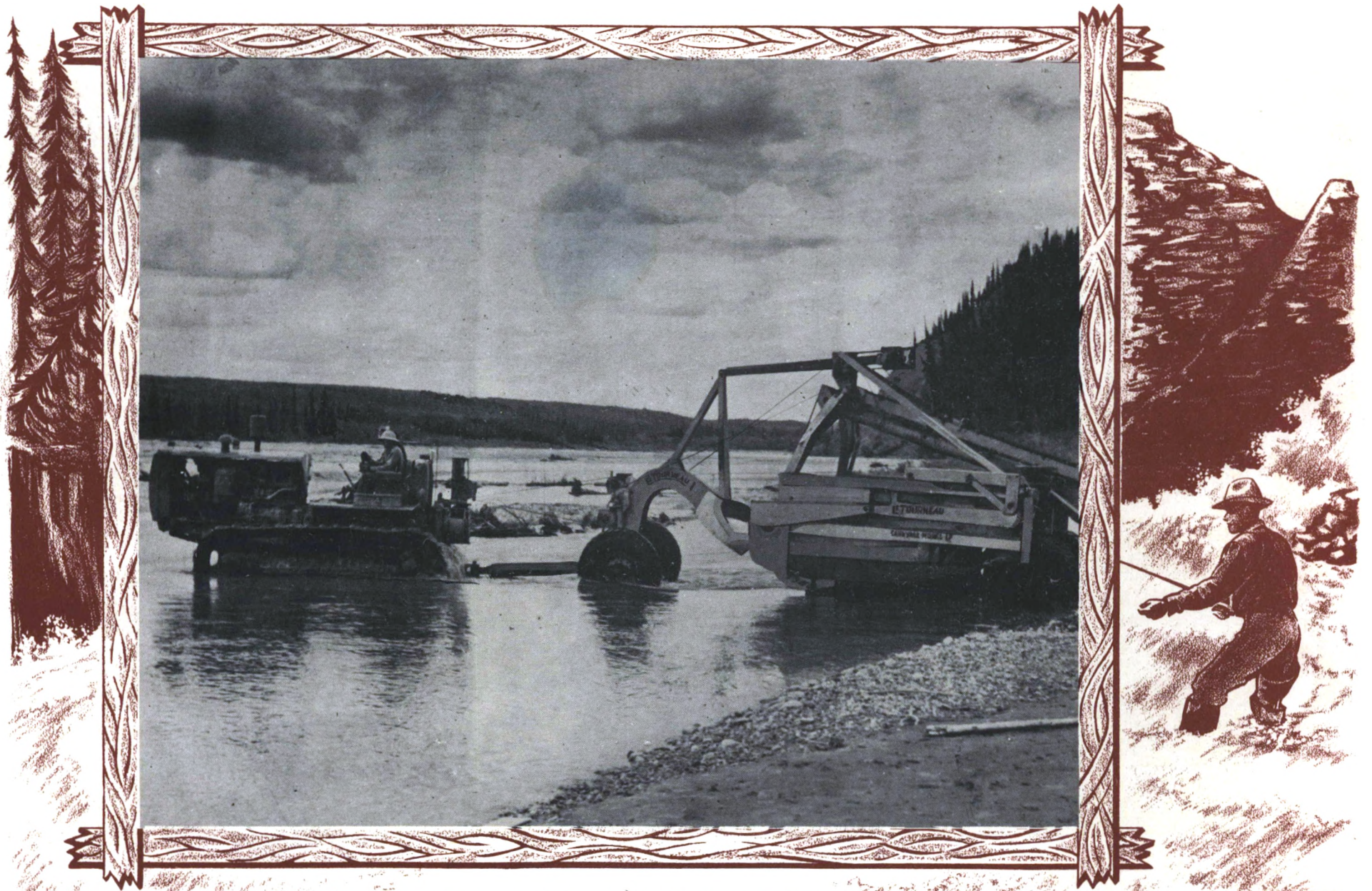
Fording one of the rivers with road-building equipment.
