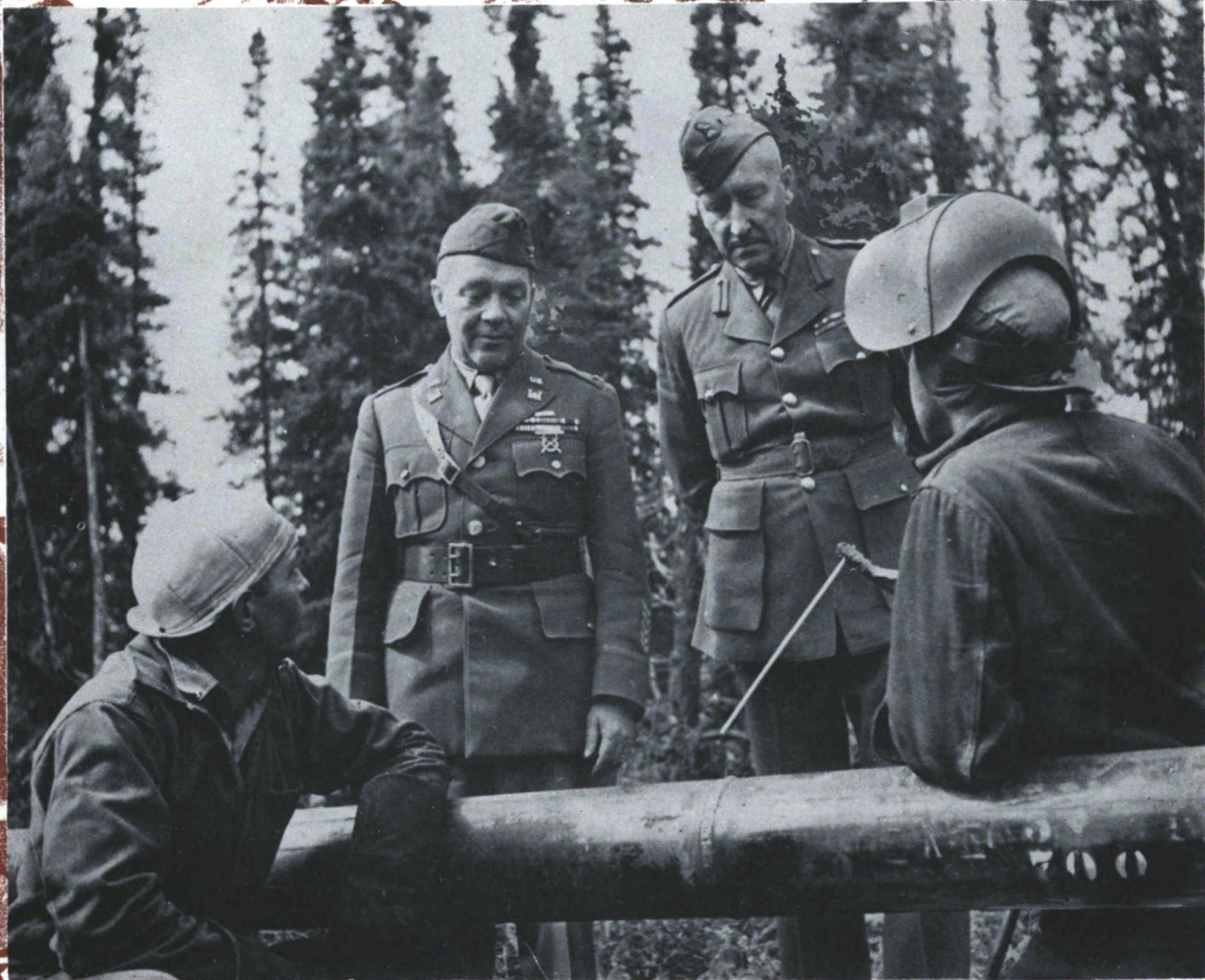
Major-General Foster, Canadian representative in the Northwest Command area, and Col. J. Lyons (left) stop to chat with welders L. S. Cook, Oklahoma, and C. R. Dunlop, San Francisco. Picture was made during General Foster's initial inspection trip.
