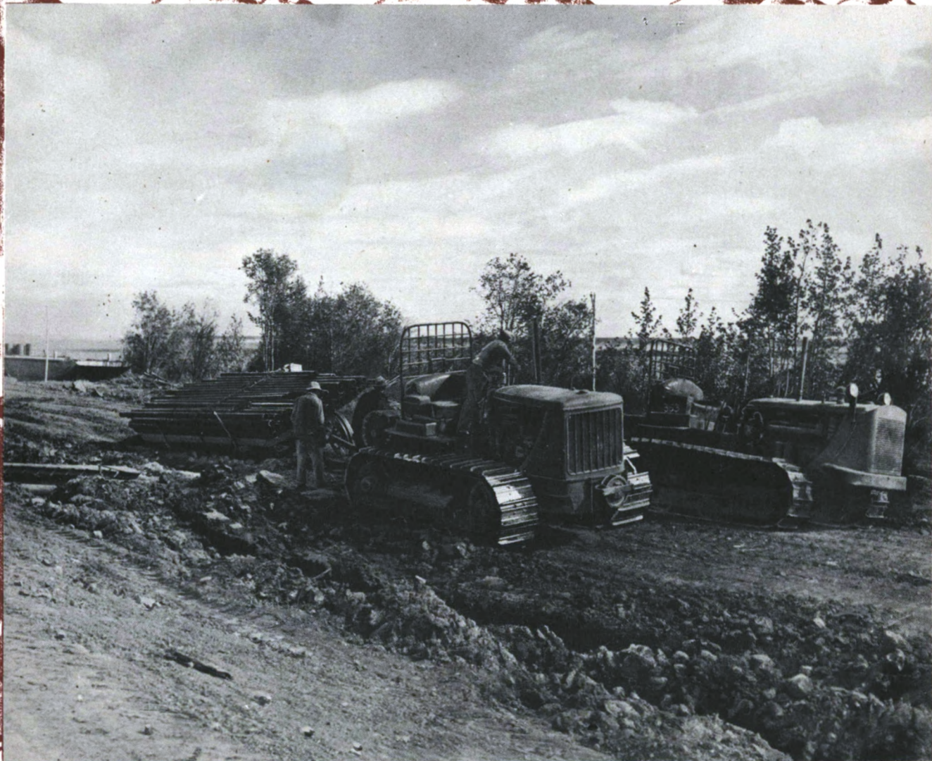
'Cat' with mutilated track receives assistance in hauling a load of pipe out of a soft spot in the road.
