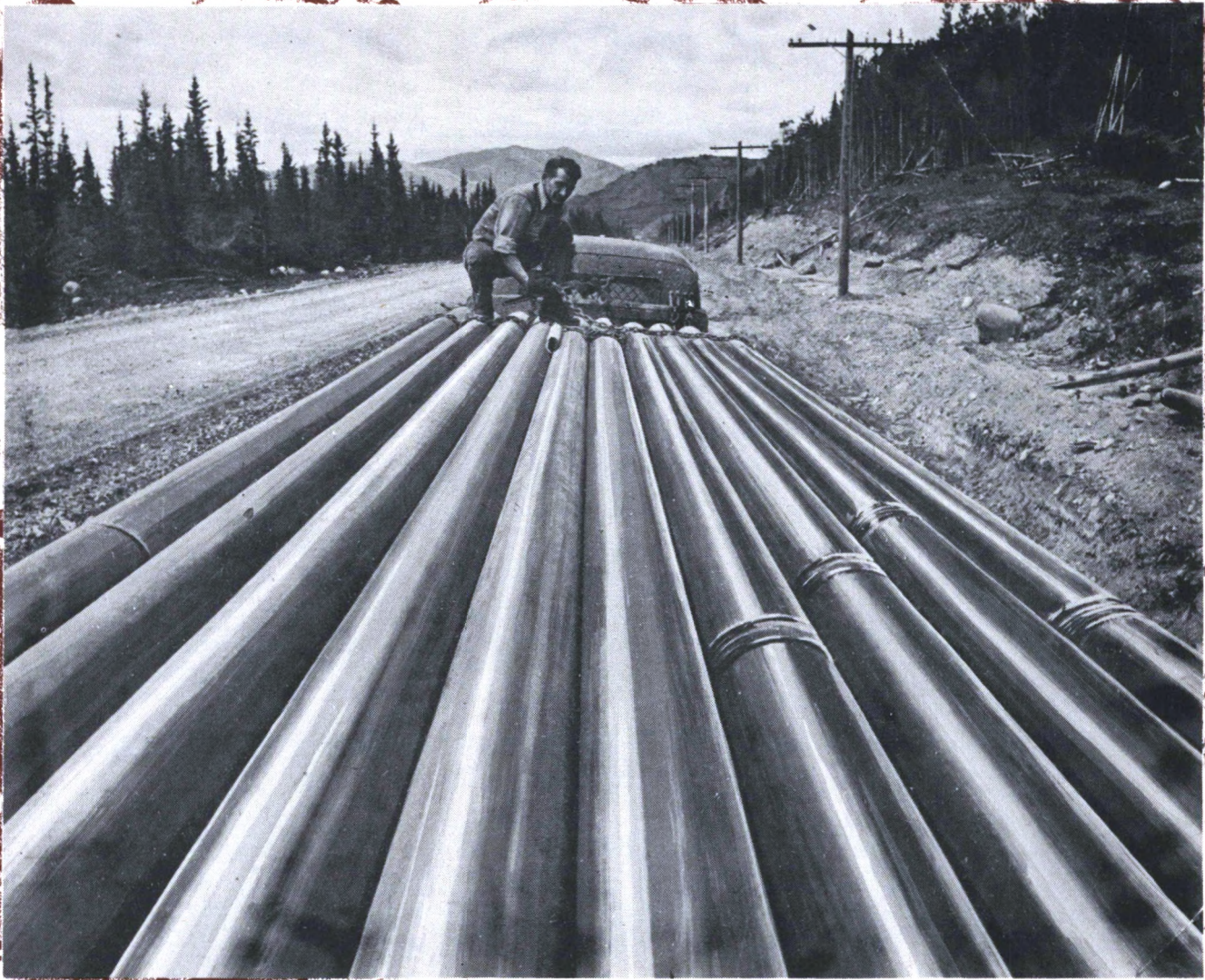
Pipe for the new pipe-line is delivered by huge trucks groaning under 7-ton loads. Here a load of pipe is being dumped. Pipe layers and welders will take over from here.
