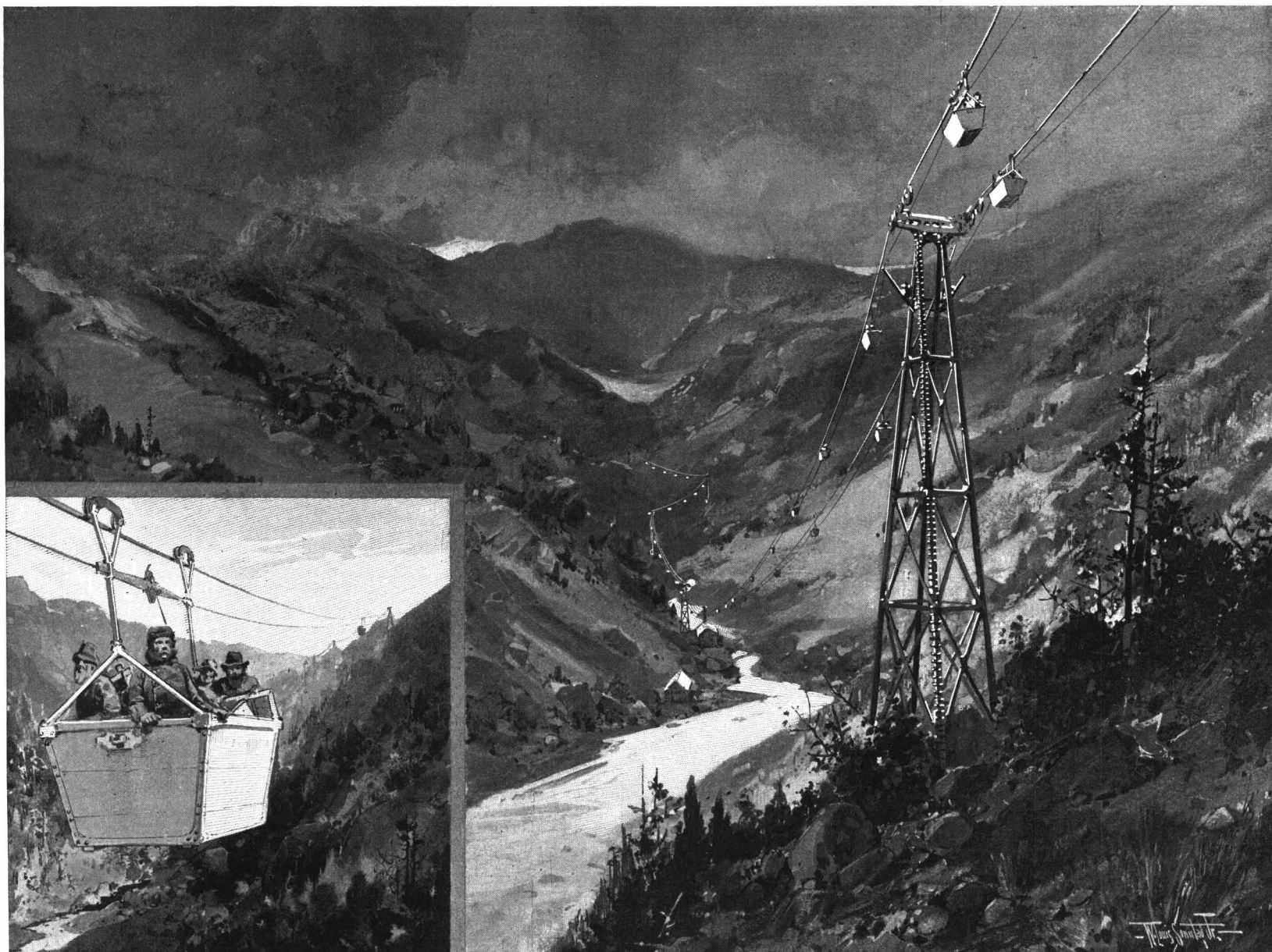
AN AERIAL RAILWAY TO THE KLONDIKE—PROPOSED METHOD OF OVERCOMING THE DIFFICULTIES OF THE CHILKOOT TRAIL.
