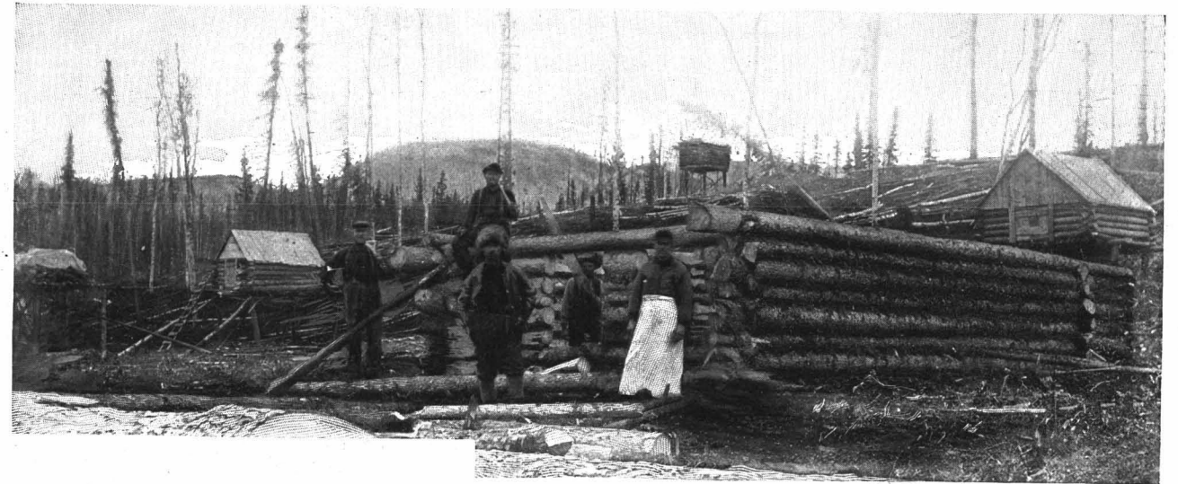
THE FIRST RESTAURANT IN RAMPART CITY IN COURSE OF CONSTRUCTION.
