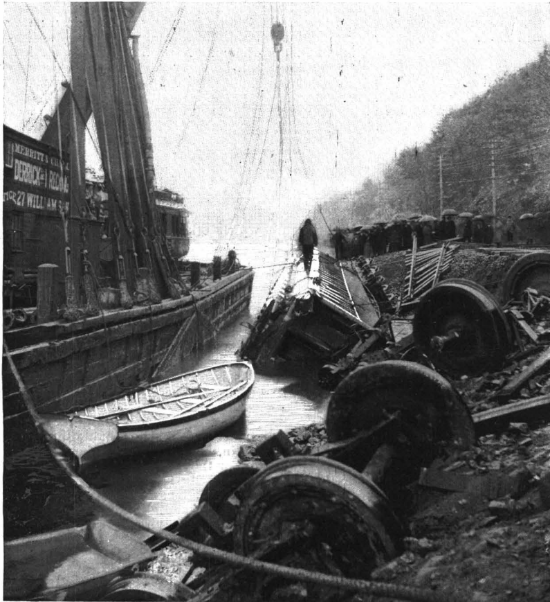
WHERE THE BREAK OCCURRED.
