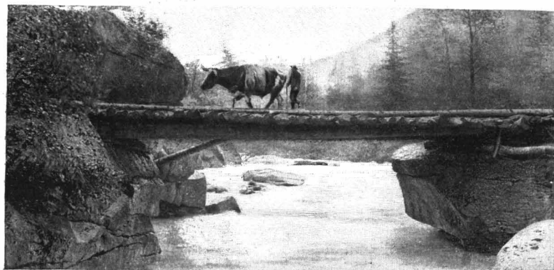
CORDUROY BRIDGE ACROSS THE SKAGWAY.
