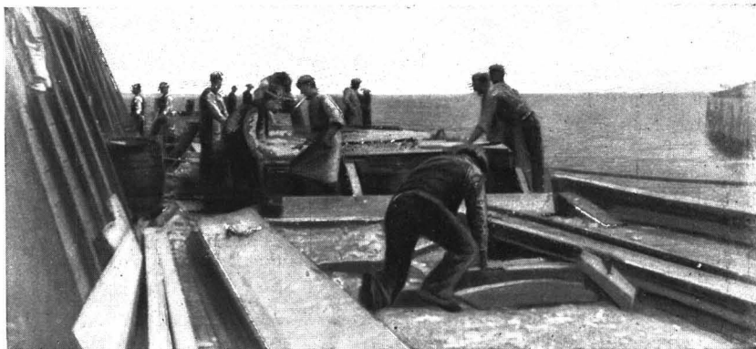
AN EVERY-DAY SCENE AT VICTORIA DOCK. Carpenters making Scows for lightering the Freight at Skagway Bay (White Pass).
