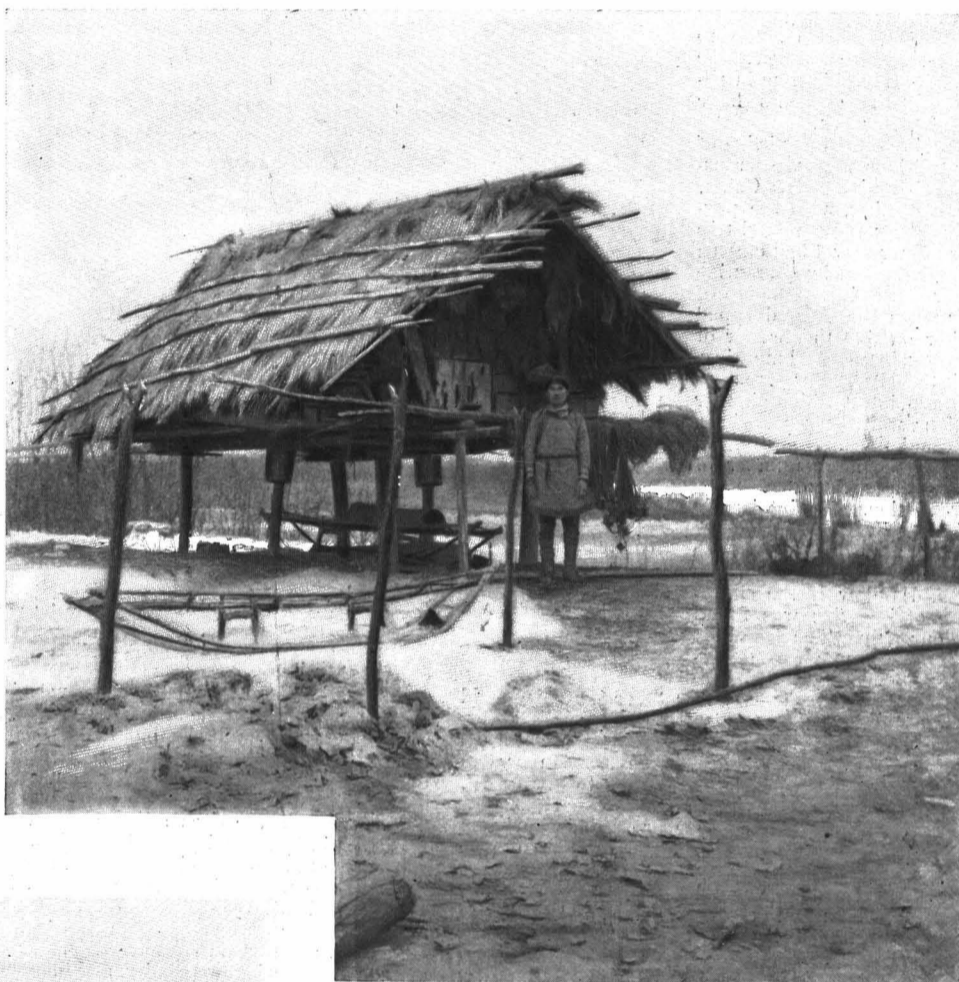
STORE-HOUSE IN A VILLAGE OF THE GOLDES. Raised on Poles to protect the Contents from the Sledge Dogs.
