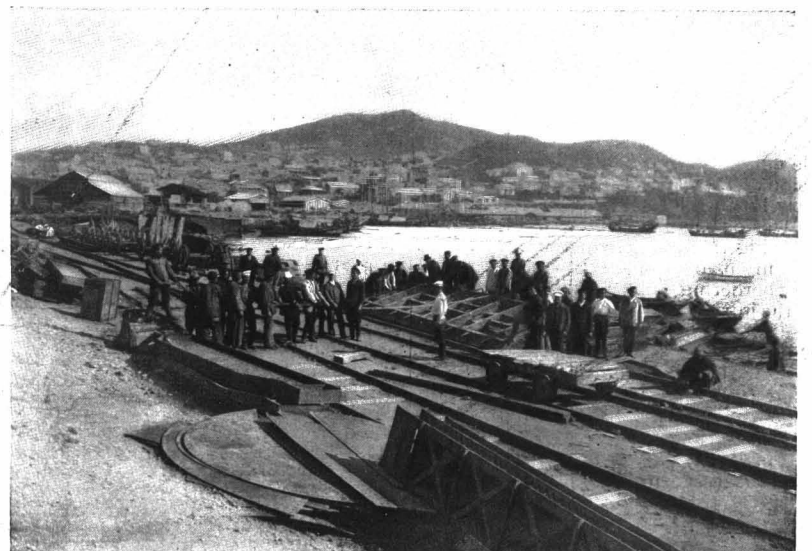
HANDLING CONSTRUCTION MATERIAL AT THE RAILWAY TERMINUS AT VLADIVOSTOK.
