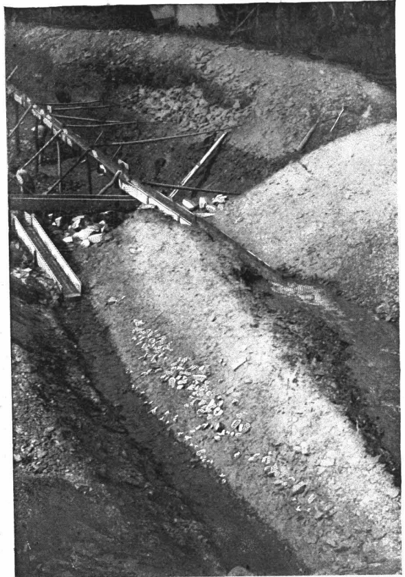
A TYPICAL PLACER CLAIM, SHOWING CUT, SLUICWAYS, AND TAILINGS.
