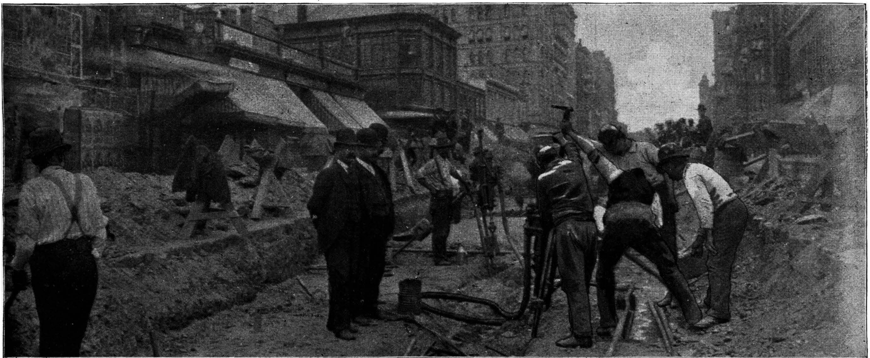
BROADWAY, NEAR THIRTY-SIXTH STREET.
