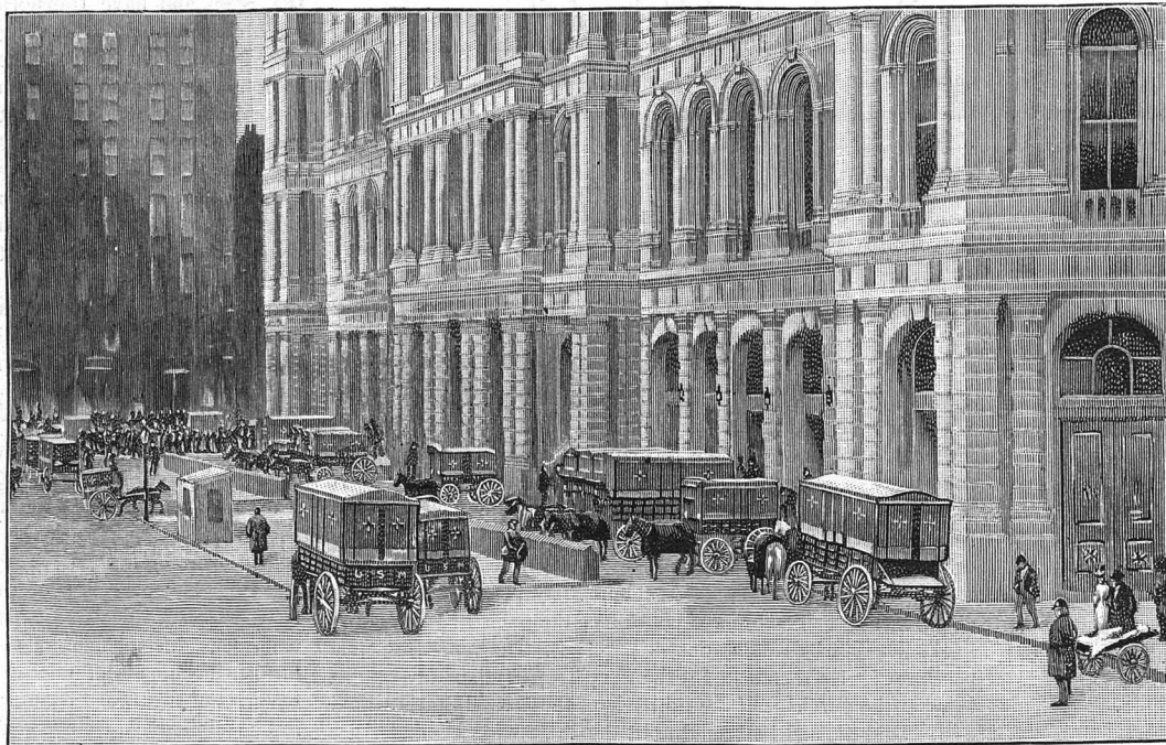
Rear of Post-Office Building, terminus of mail in bulk.
