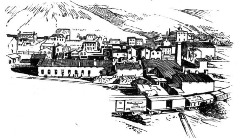
LA BELLE IRON WORKS, COOPER SHOPS.
