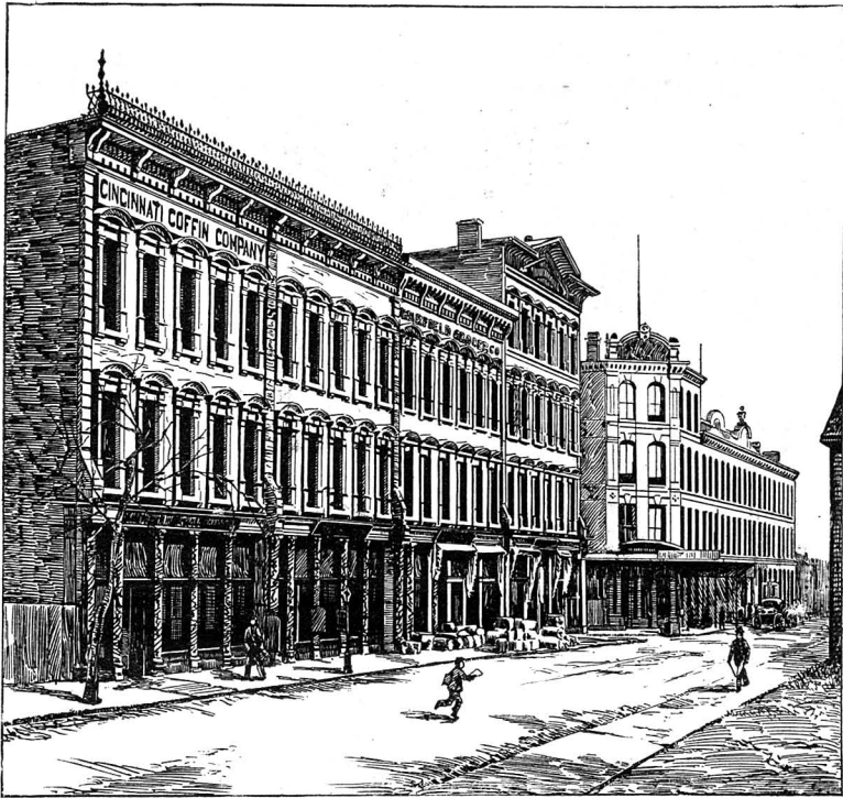
VIEW ON THIRD STREET.
