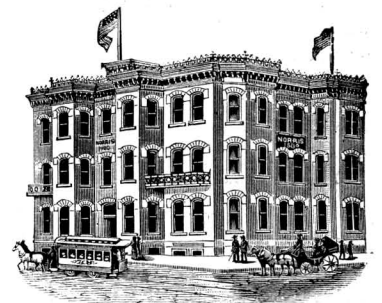
JAMES L. NORRIS BUILDING, WASHINGTON.
