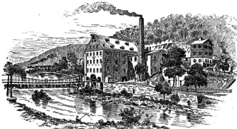
MILL "B."—PATAPSCO FLOURING MILLS, BALTIMORE, MD.
