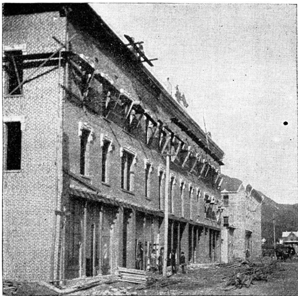
COLONNADE HOTEL, BUENA VISTA, IN COURSE OF CONSTRUCTION.
