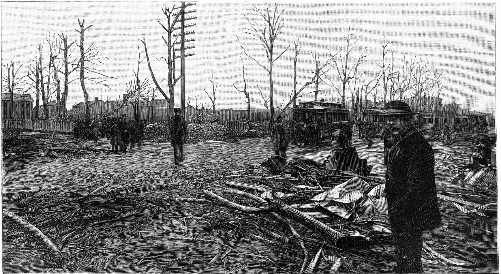
THE TORNADO'S WORK AT LOUISVILLE.—VIEW OF BAXTER PARK AFTER THE STORM. PHOTO BY KLAUBER.—[SEE PAGE 221.]
