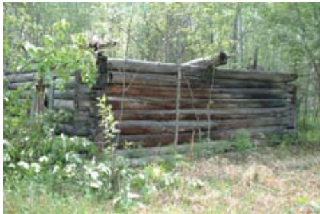
Cabin remains reported as the Alaska Commercial Company employee residence. This may be the oldest standing building at Forty Mile, dating to 1886-1887.
