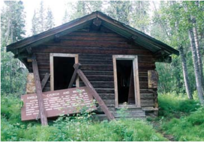
St. James church, 2000. Pieces of the interpretive sign demonstrate the effects of ice rafting. Periodic ice rafting has likely destroyed and damaged a number of historic structures at Forty Mile.
