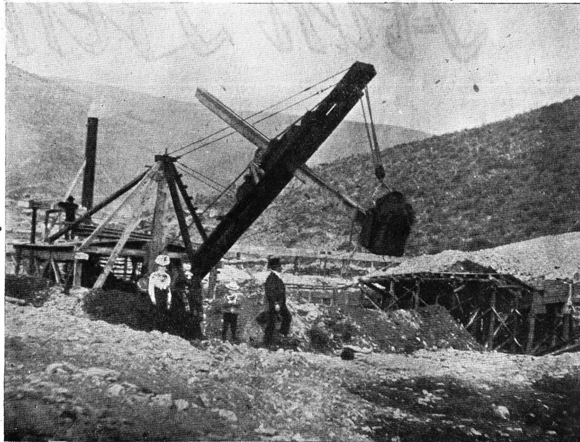
STEAM SHOVEL ON ELDERADO CREEK.
