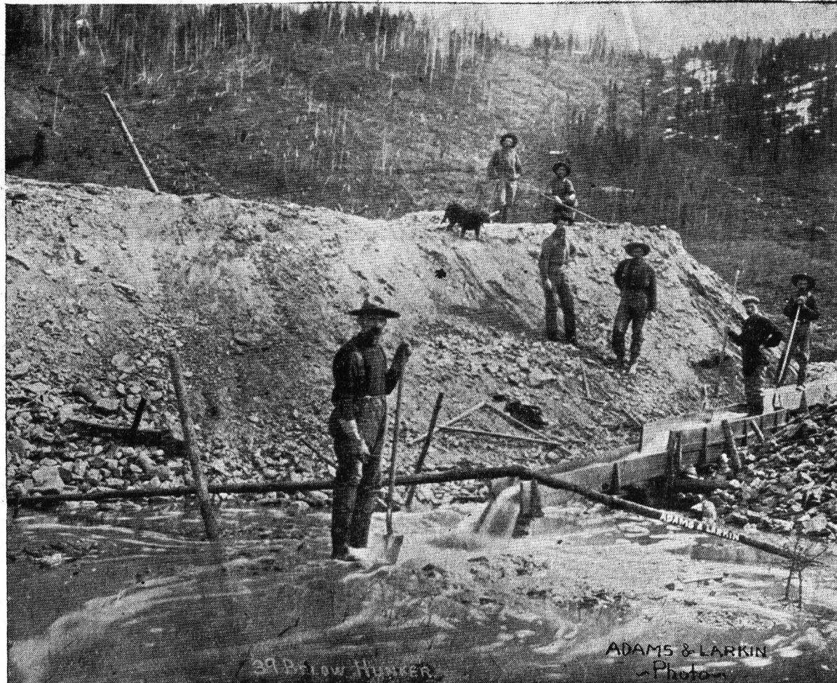
SLUICING ON HUNKER CREEK.
