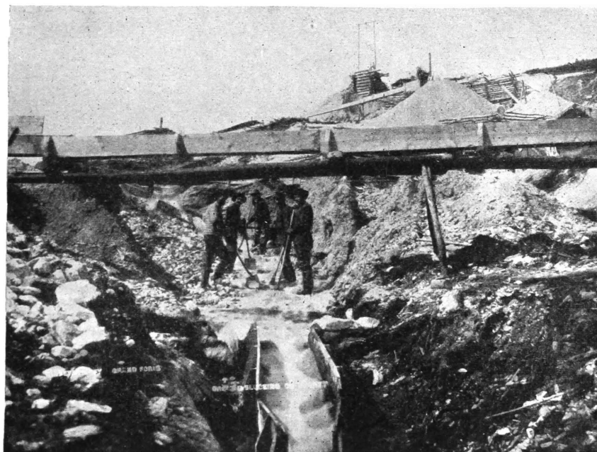
GROUND SLUICING ON MAGNET.
