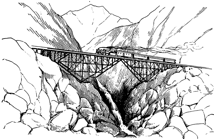
400 feet steel arch bridge at summit of White Pass & Yukon Route.
