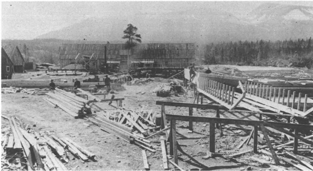
45 Exterior view, King's sawmill, Bennett, 1900. Note end walls of building on left appear to be one continuous slab, while the long side walls and the roof are larger and composed of several lengths. Building at right has walls of
