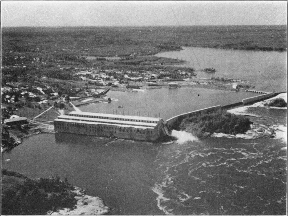
Pointe de Bois development of the City of Winnipeg on the Winnipeg River, Manitoba. 105,000 horse-power installed.
