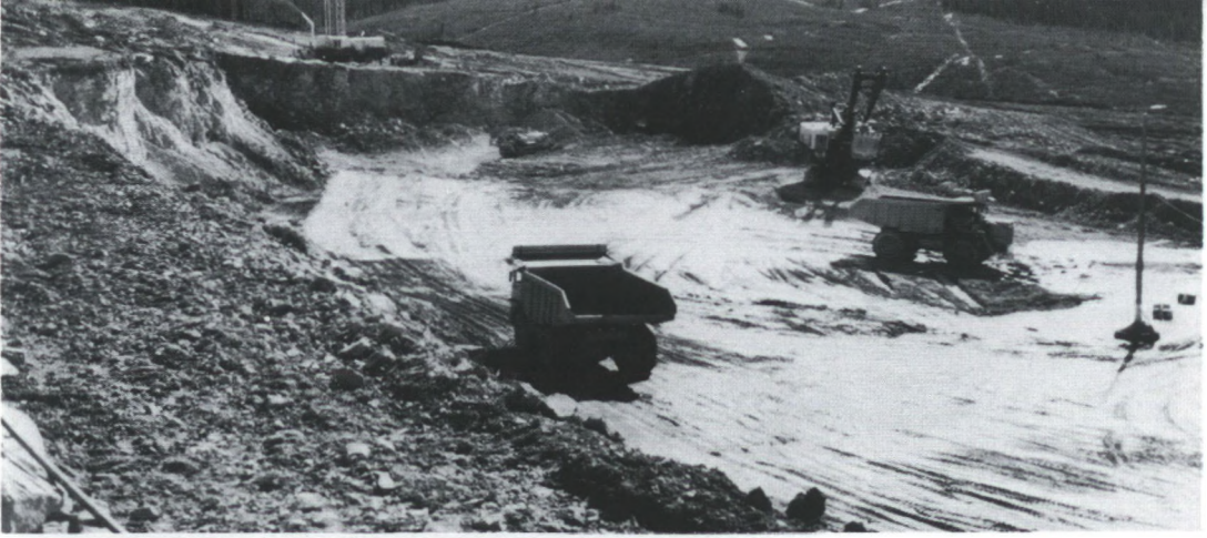
Beginning of open pit, June, 1968.
