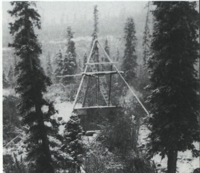
Diamond drilling to prove grade and tonnage.
