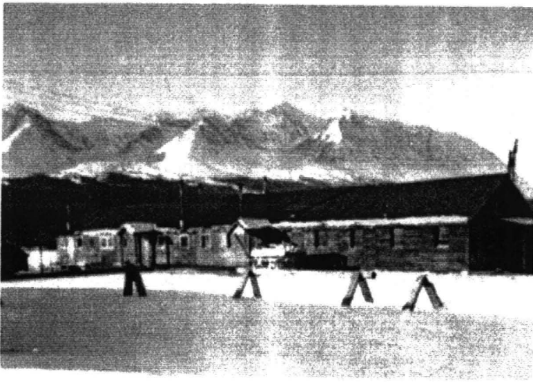
64. Haines Junction Maintenance Camp school, 1953. The senior classroom (r.) was also used as the camp recreation hall. The teachers' apartment was in the centre, and the junior classroom at the far left.
