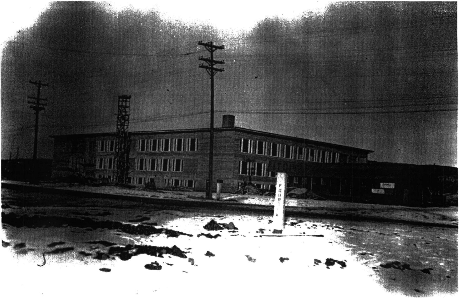
58. The new Whitehorse Elementary - High School nears completion, 1952.
