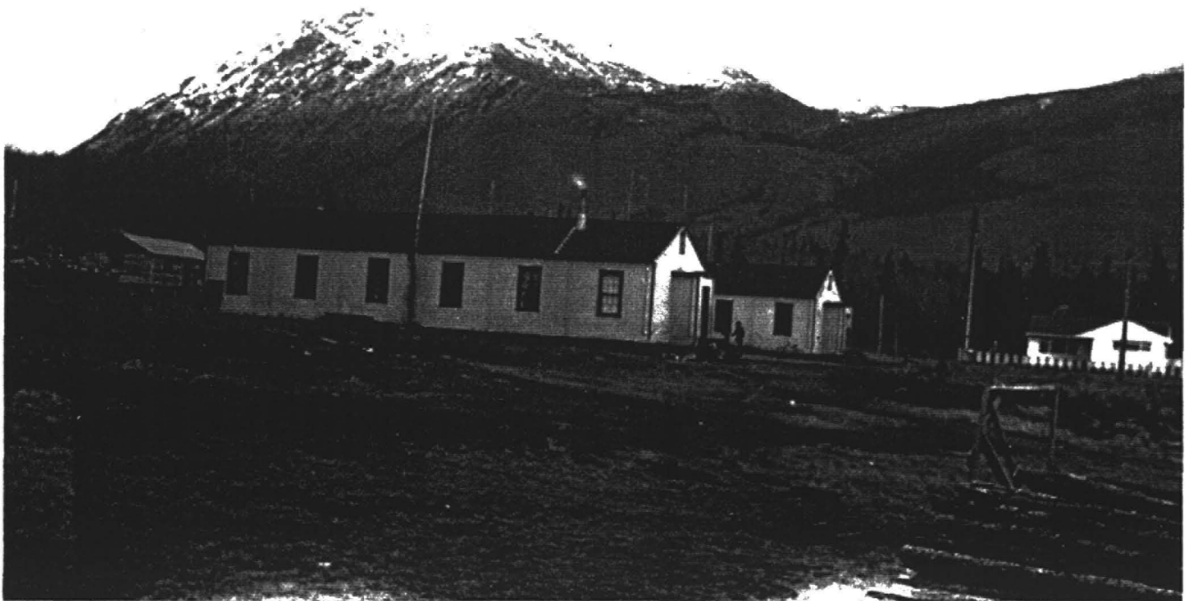
69. Chooutla School, Carcross, fall 1950. Principal's house built in 1948 is at the right.
