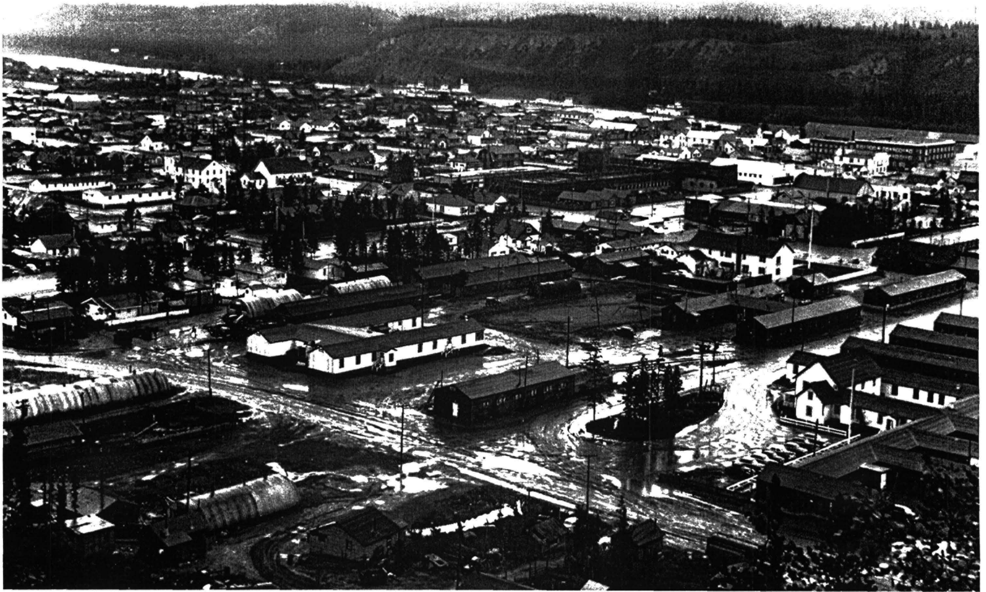
51. Downtown Whitehorse, 1953. "Federal Building" (centre) under construction; "Army" hospital buildings at lower right.
