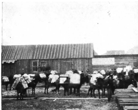
NEWMAN'S PACK TRAIN READY TO START FOR BENNETT. A TYPICAL FREIGHTING OUTFIT OF THE WHITE PASS.
