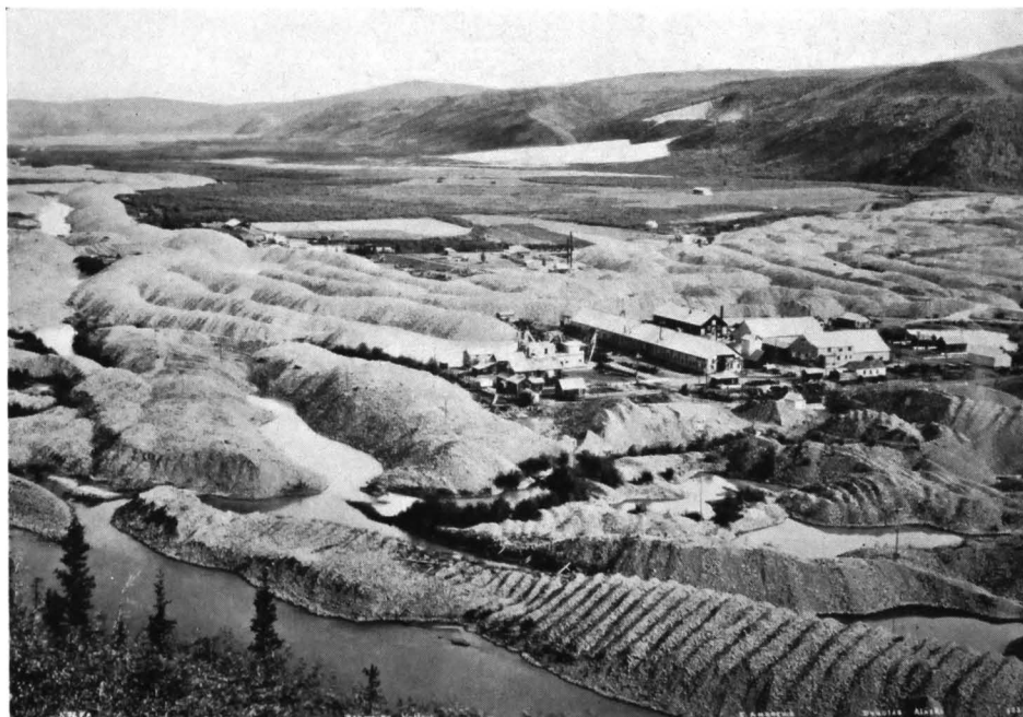
DREDGE TAILINGS ON THE KLONDIKE RIVER. MILLIONS IN GOLD ARE BEING SIFTED FROM THE GRAVEL BY THIS PRESENT-DAY MINING METHOD
