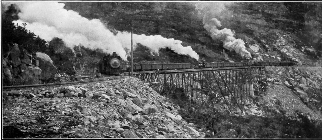
STEEL ARCH ON THE W. P. & Y. R. R.
