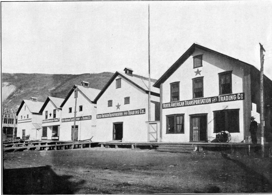
N. A. T. CO.'S OLD STORES AND WAREHOUSES, DAWSON CITY
