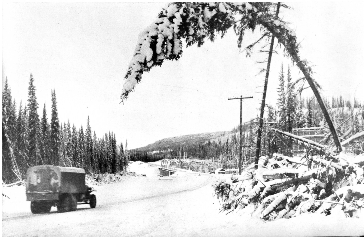
Weighted by snow, spruce tree, below, frames approach to Coal River bridge.
