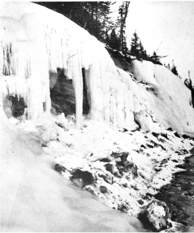
CONSTANT threat to safe operations on the Highway are glaciers forming on mountainsides adjacent to road. Molded by springs bubbling from the earth only to freeze upon reaching the surface the icy formations continually inundate sections of the Highway necessitating constant maintenance.
