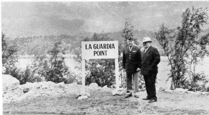
GENERAL JAMES A. O'CONNOR , Commanding General of the Northwest Service Command, and Fiorello H. LaGuardia , Mayor of New York City and a member of the joint United States and Canadian Commission that selected site for Highway, stand at point named in latter's honor.
