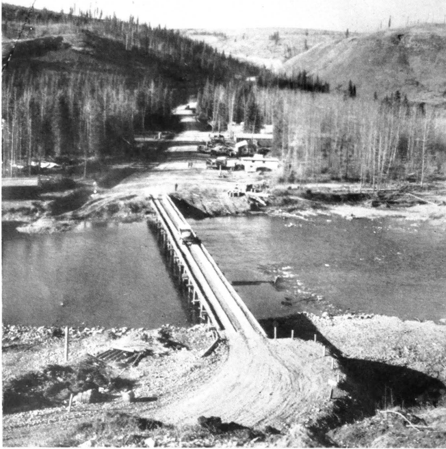
BRIDGES have played a major role in construction. Spanning the Sikanni Chief River, shown here was an easy task for Army.
