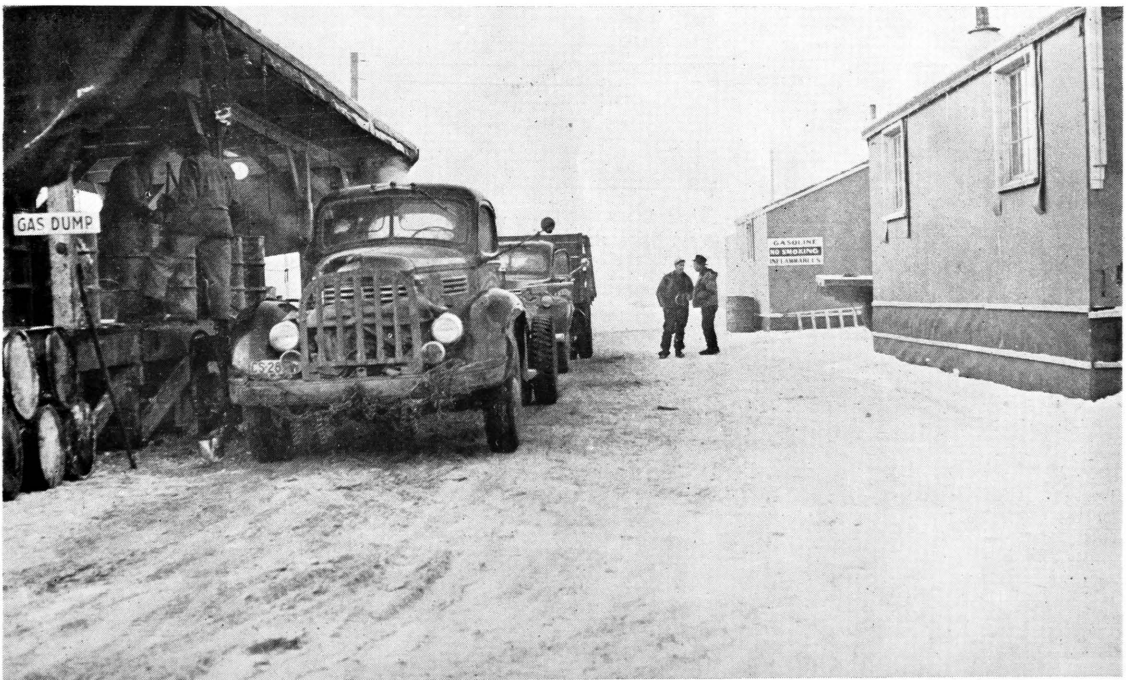
FUELING station at Fairbanks is a key point of the station's operation. Covered gas dumps, as illustrated, have mostly given way to underground storage tanks with self-computing pumps. At first dumps did not even have covers.
