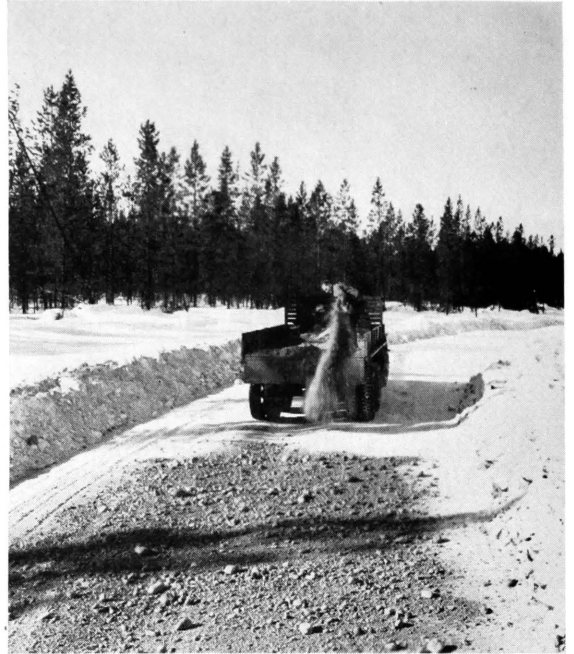
CREWS OF maintenance men, busy during the summer months improving the Highways are employed as soon as the snows begin to cover the terrain in sanding icy sections of the road. Curves, grades and bridges are kept safe for travel by frequent applications of gravel.
