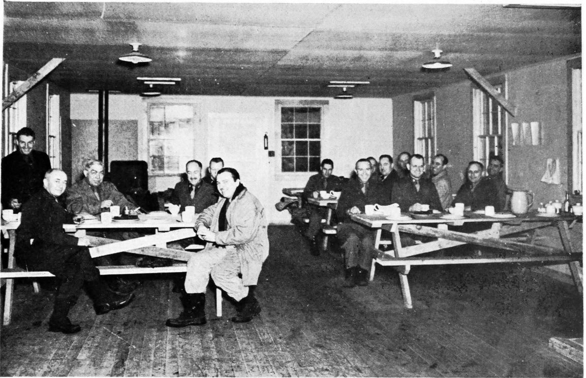
MESS HALL is visited by Army and governmental officials travelling up the Alaska Highway. Seated at table, extreme left,
