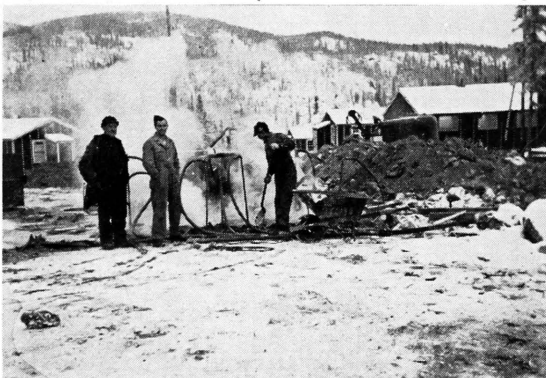
Construction activities in camp area.
