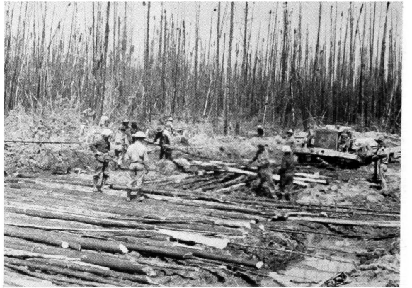
TO WHIP the muskeg, corduroy roads were laid over the mucky earth. Below: At 50° below, they hung an icy wash on the line.
