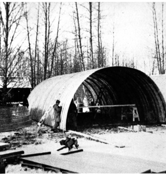
TROOPS arriving on the Highway lost little time in making themselves comfortable. Buildings of the type shown above were rapidly assembled by the men. This type is particularly adaptable for use in Arctic regions; due to its rounded architecture it is able to withstand gales and drifts of snow.
