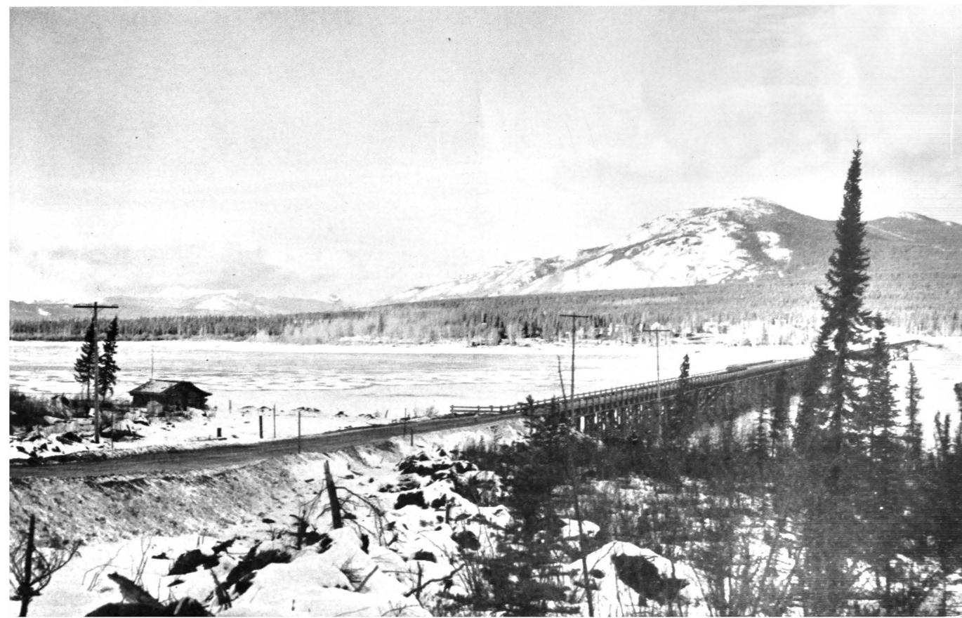
Scene below shows Teslin Lake with pile-type bridge and trapper's cabin.
