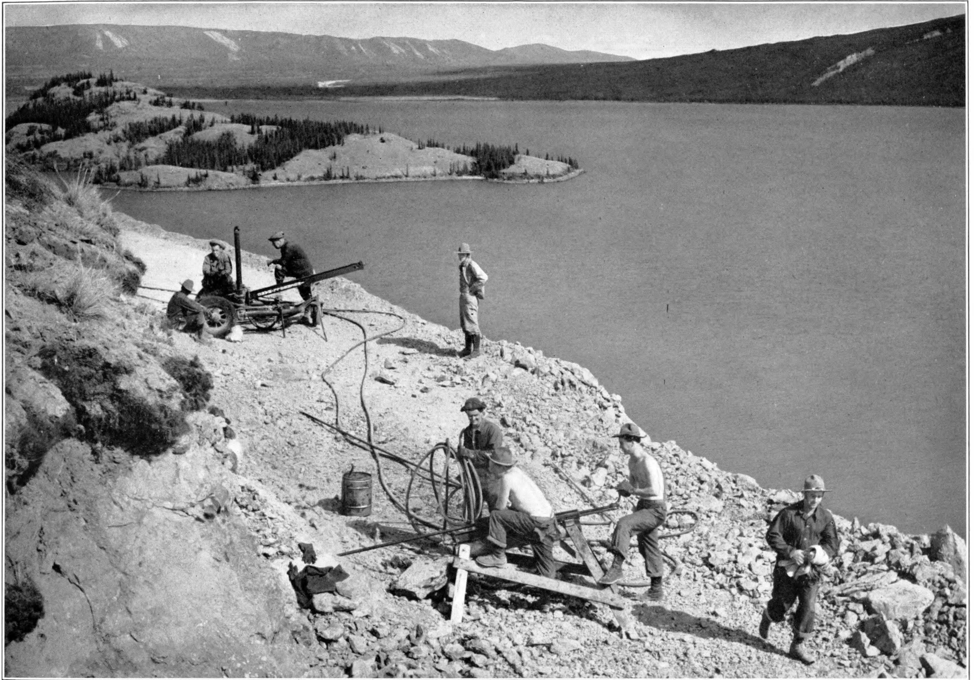
Pneumatic drilling device at work over a high piece of the Alcan Route in the Yukon.
