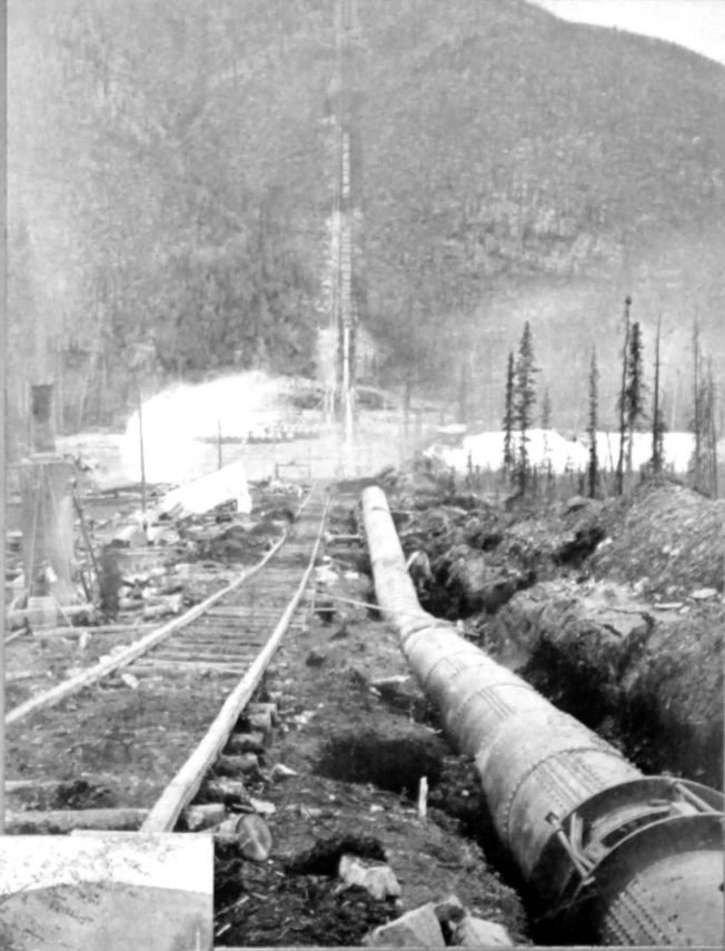
Pipe line under construction crossing Little Twelve-Mile River, taken from above the Power Plant.
