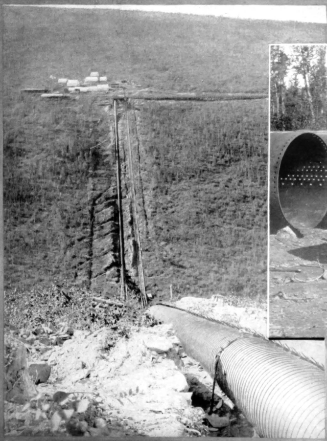
Wood stave pipe crossing on Bonanza Division.
