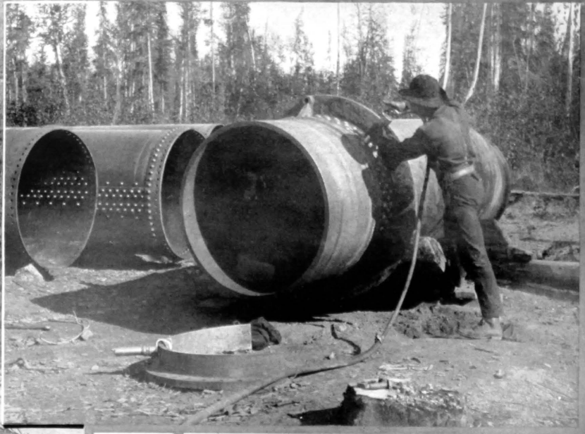
Rivetting expansion joint, Klondike syphon.
