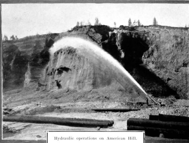
Hydraulic operations on American Hill.
