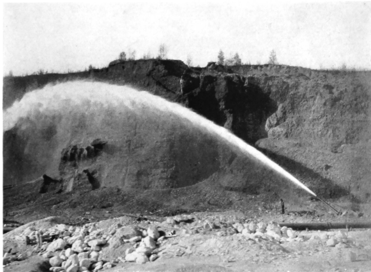
HYDRAULICKING ON AMERICAN HILL.
