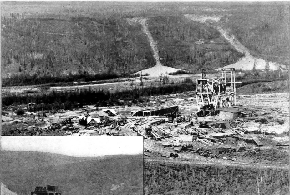
Dredge construction at mouth of Bonanza Creek,—two dredges building in the same pit. Shows one dredge complete to the superstructure and the hull of the other under way. Note hill deposits and hydraulic tailings in the background.
