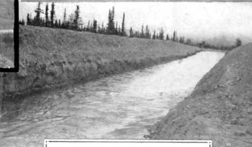
Finished ditch in operation.
