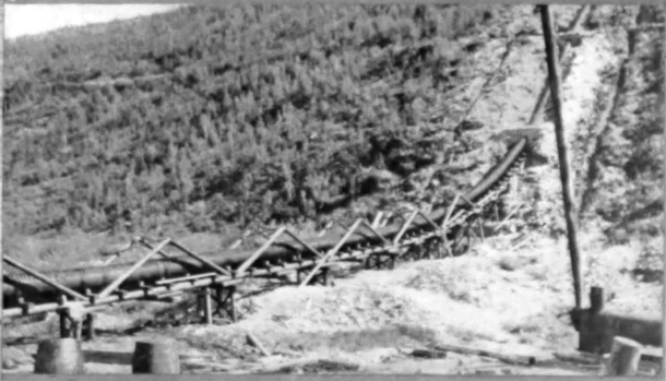
Portion of the Bonanza Division, showing pipe line crossing Adams Creek.
