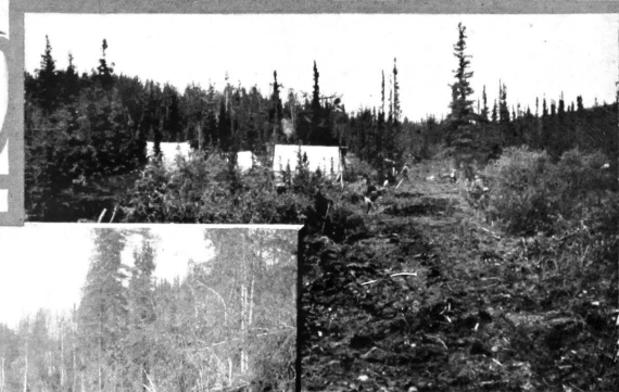
Road construction. Clearing right-of-way.
