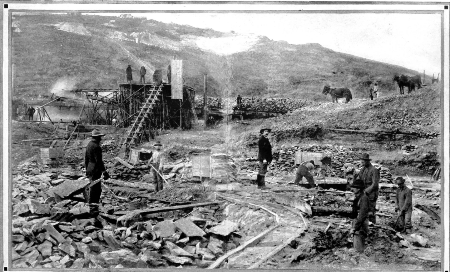
OPEN CUT ON BONANZA, SHOWING EARLY METHOD OF TRAMMING AND WASHING. NOTE THE HIGHER LEVEL OR "WHITE CHANNEL" DEPOSIT IN THE BACKGROUND.
