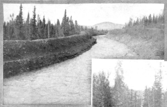
Main ditch in operation.
