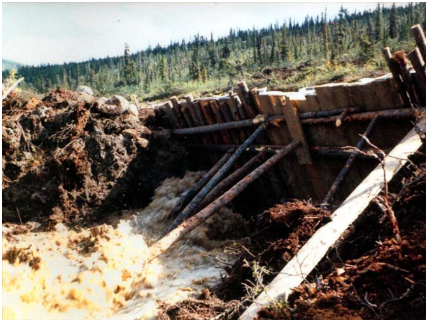
First sluice dam, about to collapse ca. 1974 YA 2003/05 #08
