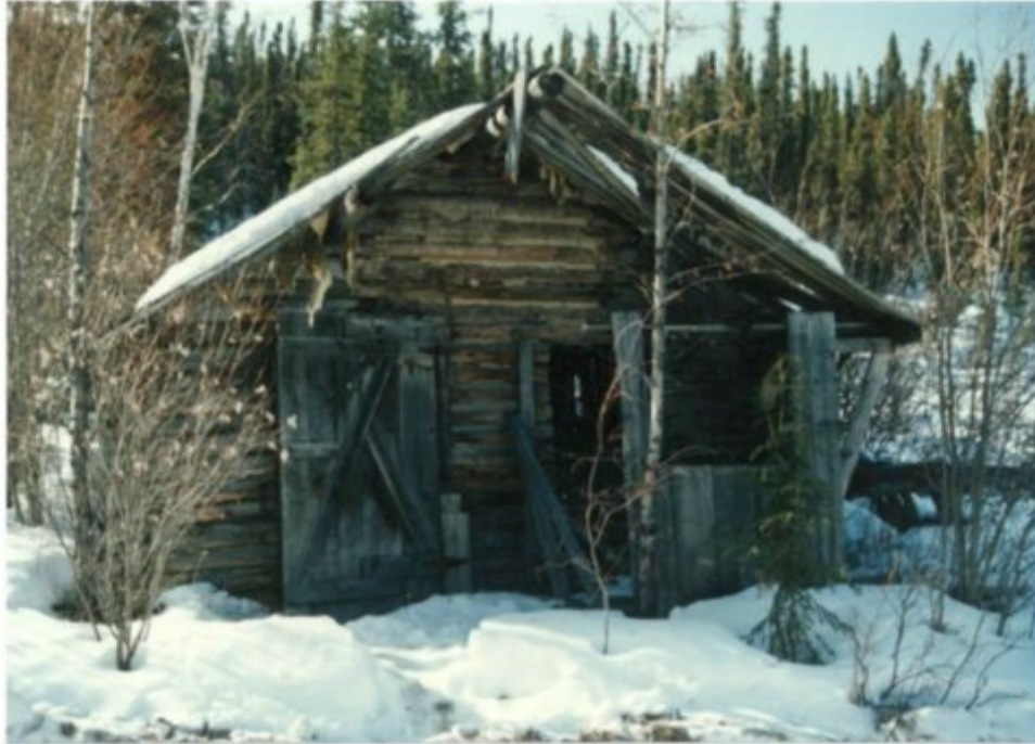
Tool Shed (Work Shop) Built by Tom Kerruish. Photo by Saugstad, 1993, for DIAND
